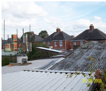
Solar Panel ("wind turbine" previously removed)
